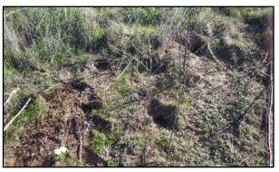
**Animal Burrows:** Animal burrows into the levee slope may allow for a preferred path for floodwater. An effective animal control program can help reduce the risk associated with borrows.
