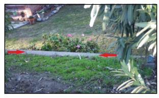
*Encroachments:* Unpermitted encroachments, such as the retaining wall shown above that cuts into the levee prism, have not been evaluated to determine the potential to negatively impact the levee.
