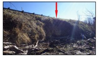
*Erosion of Levee Slopes:* The waterside earthen levee slope has eroded at different locations, likely as a result of river flows. Repair of the slope and placement of slope protection, such as riprap (rock), may protect the slope from additional erosion.
